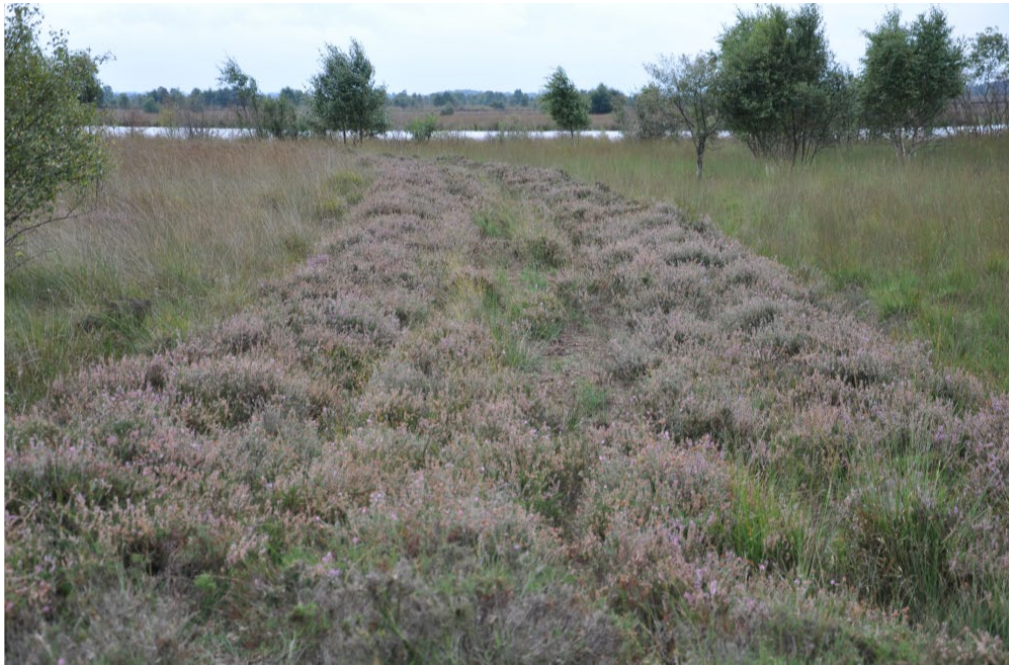
Figure 1a. Dike in Bargerveen separating the nature reserve into hydrological compartments. The dike surface is relatively dry and covered by Vaccinium dominated vegetation in mid-September 2012. To the left and right peatland is in restoration. In the background the open water reflects an earlier stage of restoration. Photo by Henry Hooghiemstra.
